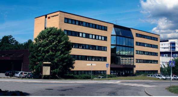
Terco headoffice and factory outside Stockholm, Sweden
